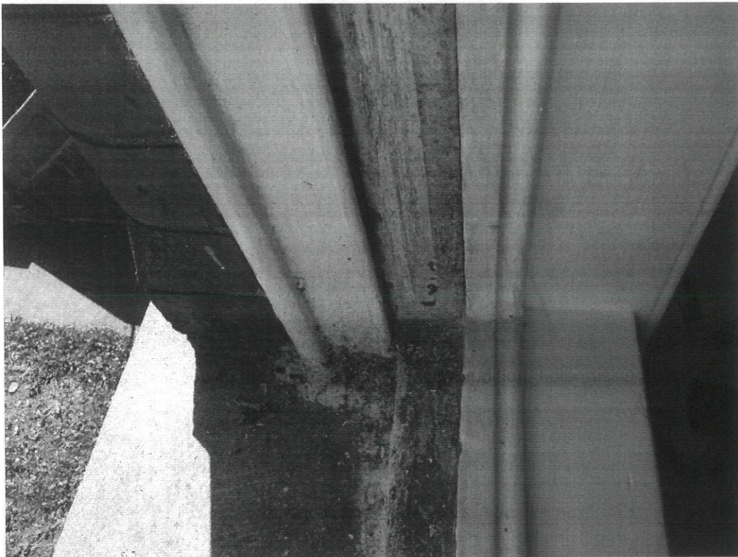
Photo 4 – Typical window sill to the front, generally good condition
